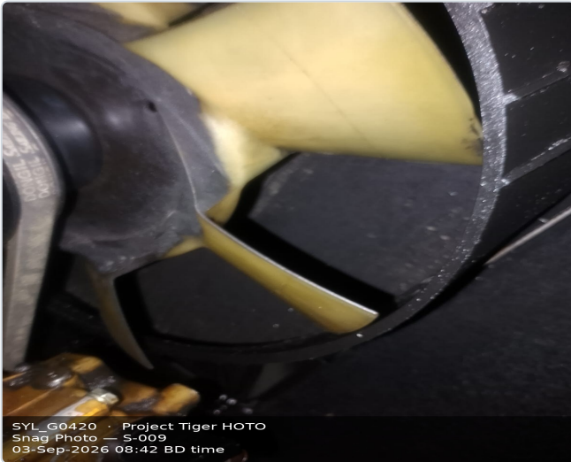
Photo 4 — S-009 — Radiator fully block dust
